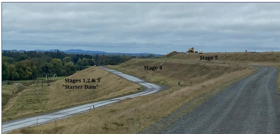
**Plate 13.1: Existing embankments side profile (provided by the client)**
